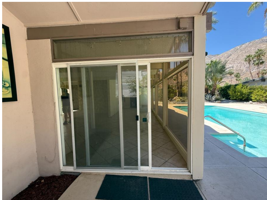
Figure. Detail view of sliding aluminum-framed glazing inserted within the former open rear patio bays. Photograph by author, 2026.
