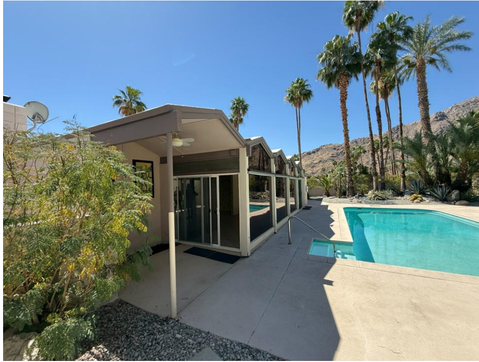
Figure. Existing enclosed rear patio addition viewed from the pool terrace, showing the incorporation of aluminum-framed glazing beneath the original folded-plate roof forms. Photograph by author, 2026.
