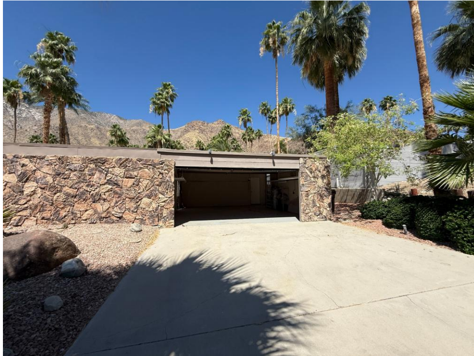
Figure. Existing condition of the primary façade and garage court of the Martin Residence, showing the broad stone-clad street wall and open garage bay. Photograph by author, 2026.
