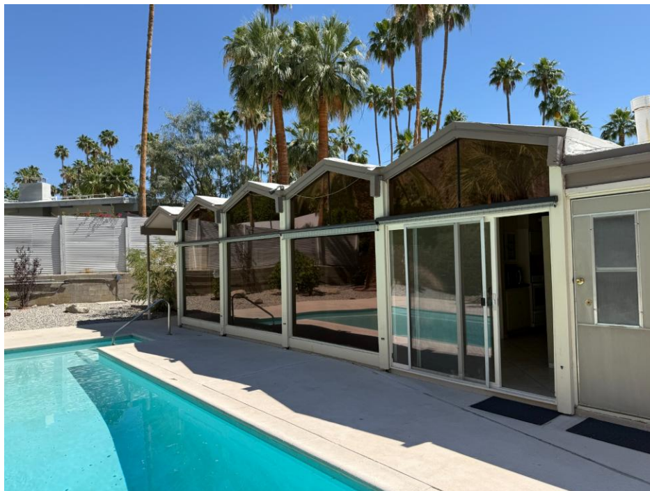
Figure. Oblique view of the rear elevation showing the rhythm of folded-plate roof forms and dark-tinted glazing added within the original patio opening system. Photograph by author, 2026.
